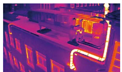
Temperature monitoring for building thermography
