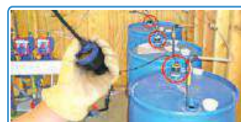
Municipal Chemical Feed Tank Tank Liquid Level Sensor
