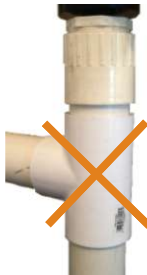
Avoid the use of a tee within the stand pipe. A tee can create false signals that will negatively effect the sensor's performance.
